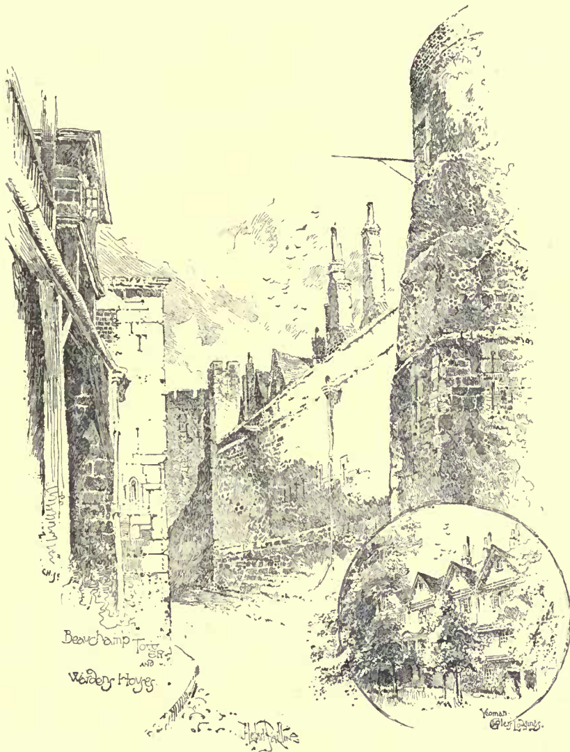
BEAUCHAMP TOWER, WARDERS' HOUSES, AND YEMAN GAOLERS' LODGINGS: TOWER OF LONDON.
