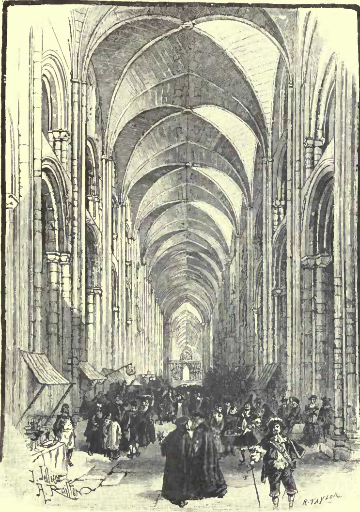
INTERIOR OF OLD ST. PAUL'S.
